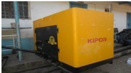
A 35KVA generator to be connected to three of the boreholes that supply water to the hospital
