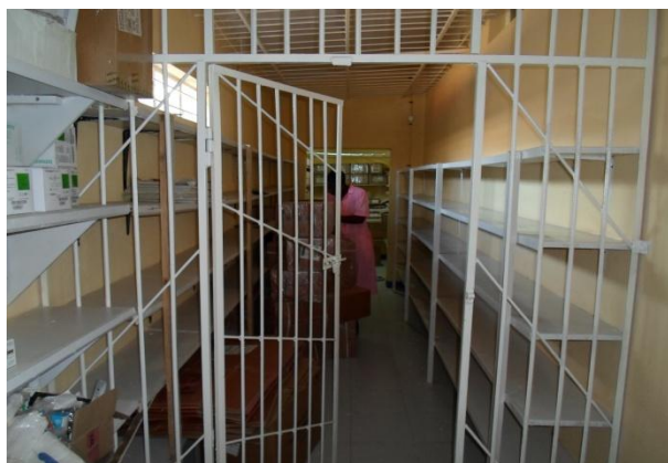
Inside the pharmacy department after the renovation, tiling, fitting of screen for securing ARVs and fitting of new shelves
