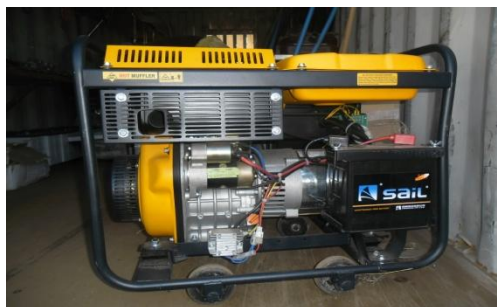
10 KVA generator to be connected to maternity dept
