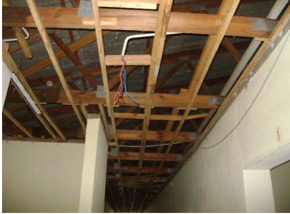
Removal of all the ceiling
